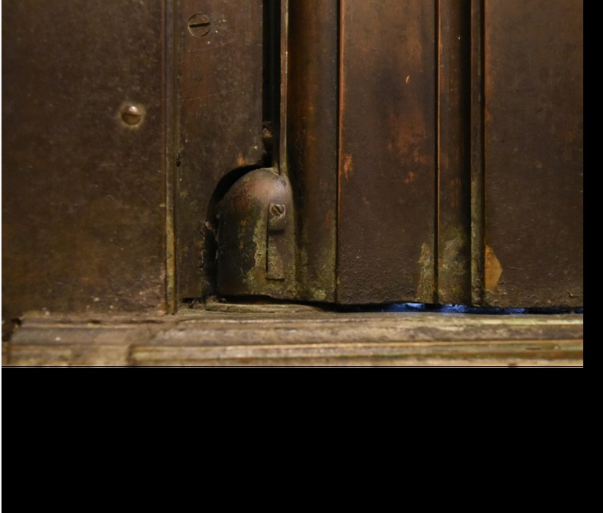
Fig. 6, Detail, inside bottom left corner of Morgan doors showing custom-fit bronze cap to cover peg on door, Morgan Library, New York. [return to text]
