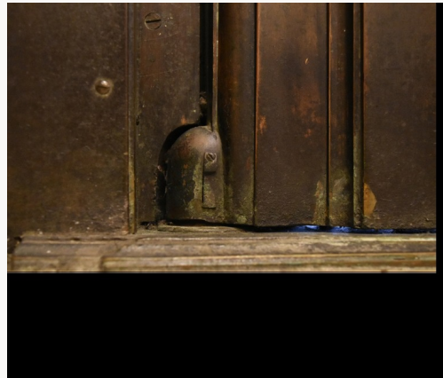
Fig. 6, Detail, inside bottom left corner of Morgan doors showing custom-fit bronze cap to cover peg on door, Morgan Library, New York. [view image & full caption]
