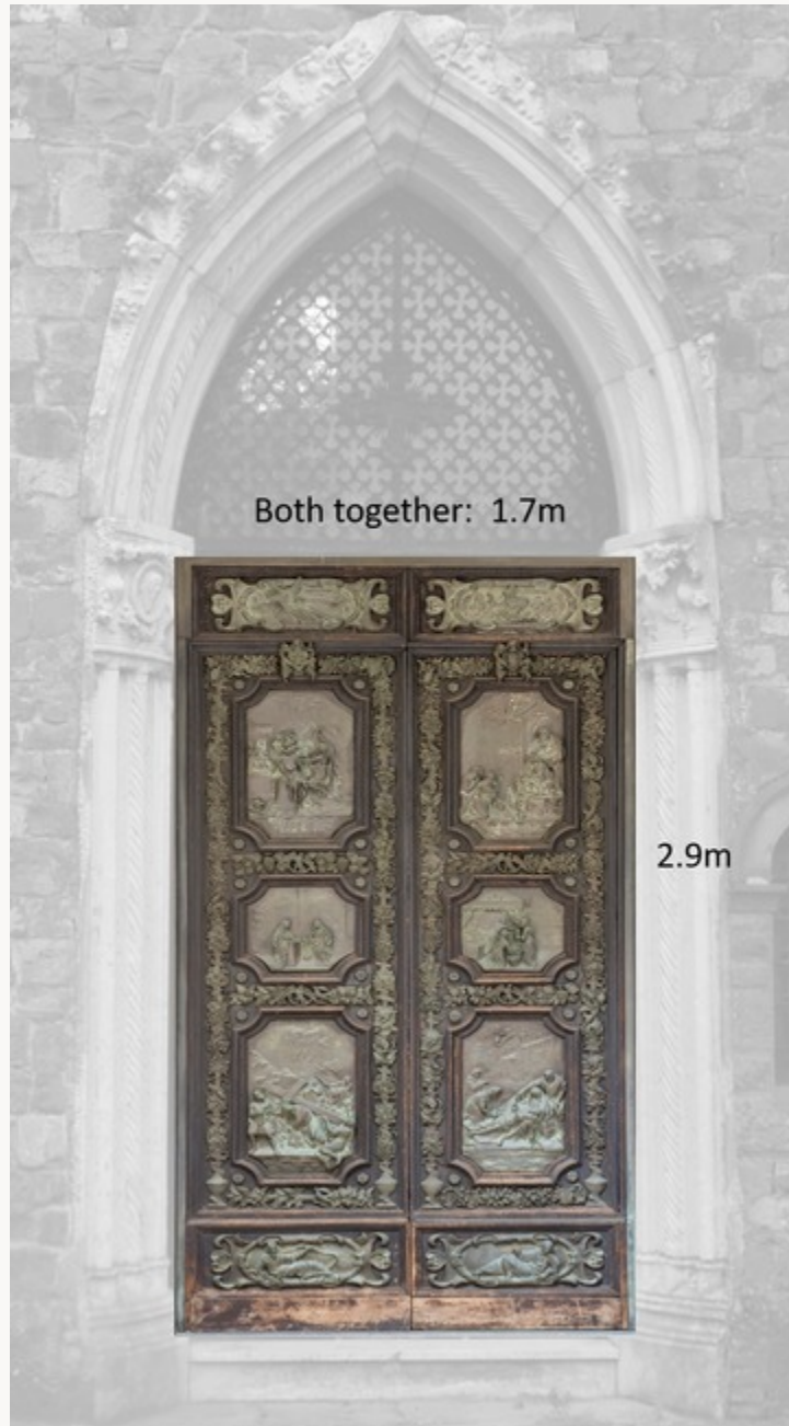
Fig. 3, The dimensions of the door as measured from the inside are as follows: left-hand door, 114.25 x 34 in. (2.9 x 0.8636 m.); right-hand door, 114.25 x 33 in. (2.9 x 0.8382 m.). [return to text]
