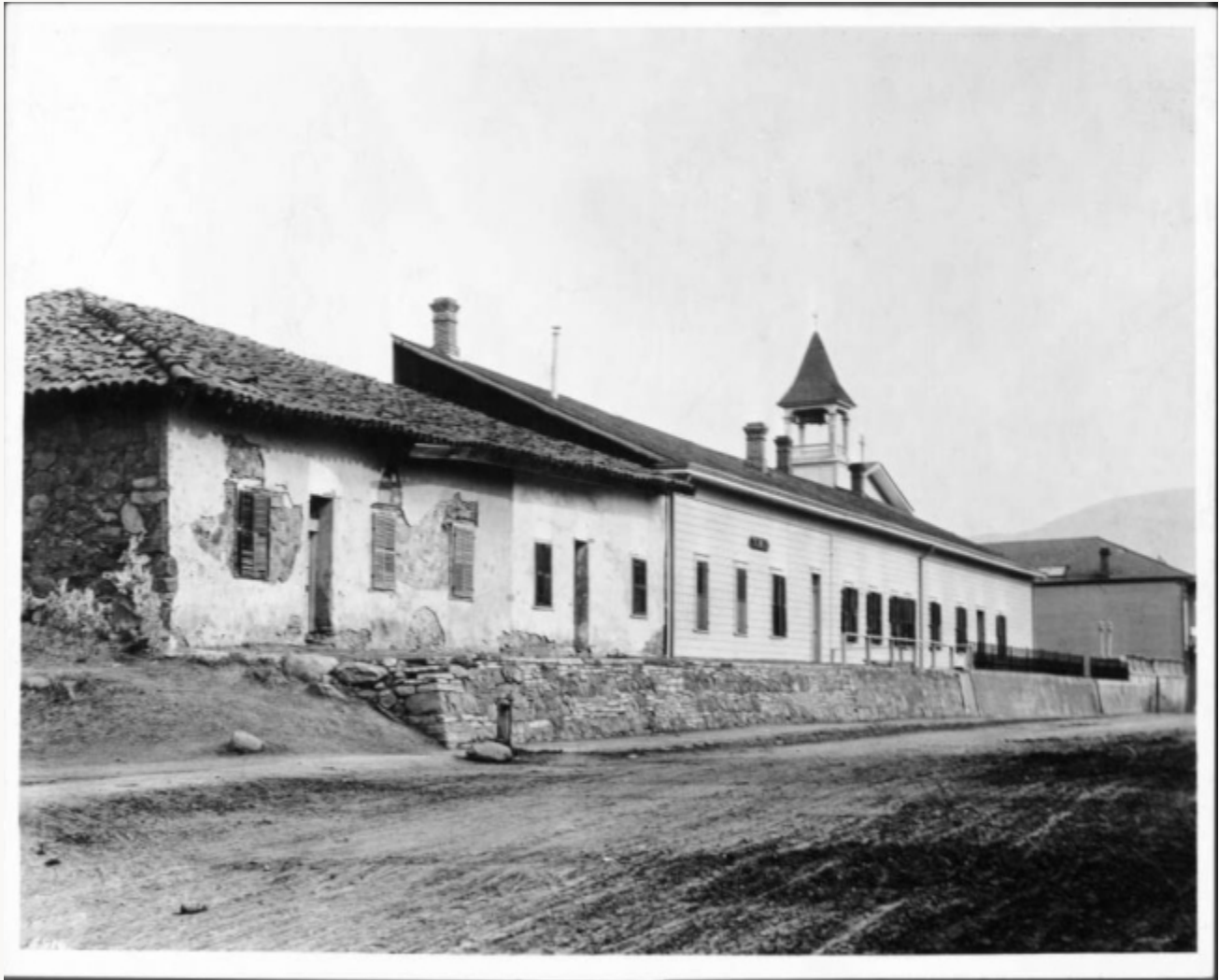
Fig. 20, C. C. Pierce, Exterior of Mission San Luis Obispo de Tolosa showing the south wing, San Luis Obispo, California, ca. 1900. Photograph. California Historical Society Collection, University of Southern California Libraries, Los Angeles. Artwork in the public domain; available from University of Southern California Digital Library, http://digitallibrary.usc.edu/ . [return to text]
