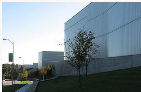
Fig. 2, East elevation of Bloch Building. [larger image]
