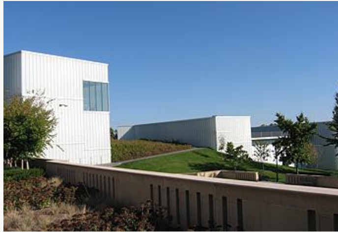
Fig. 3, West elevation of Bloch Building as viewed from front terrace of the Nelson-Atkins Museum of Art. [return to text]
