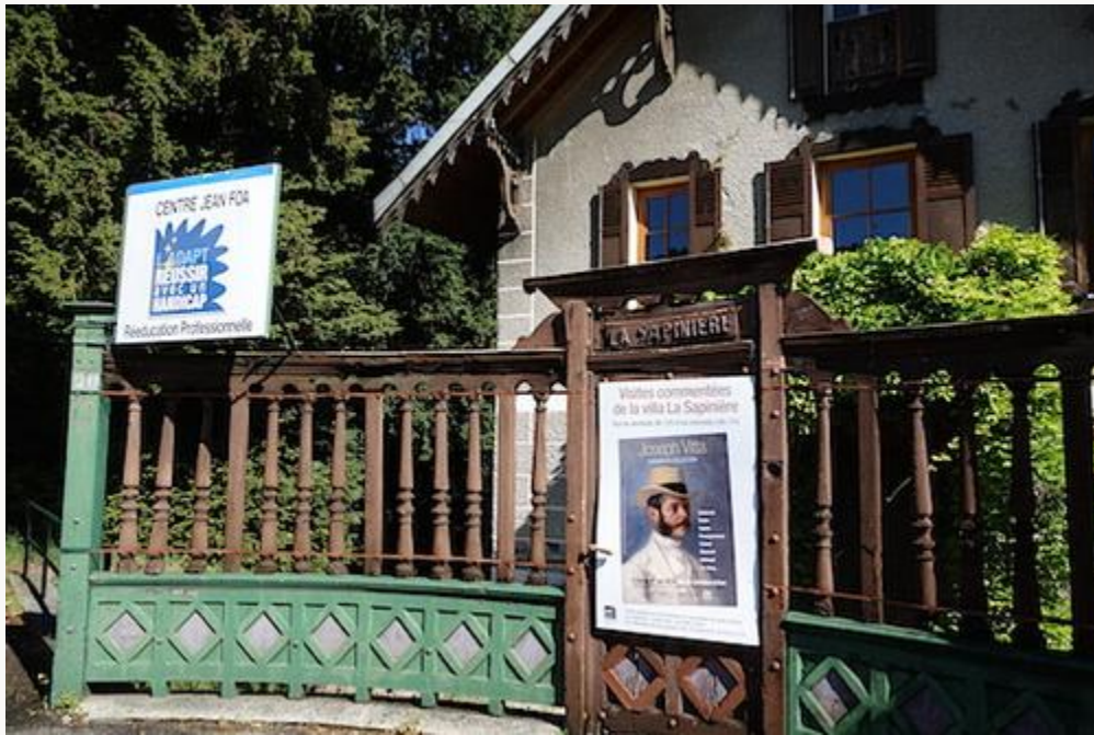
Fig. 26, La Sapinière: Gate house. [return to text]
