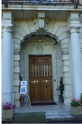
Fig. 30, La Sapinière: Jean-Camille Formigé, Main entrance. [larger image]
