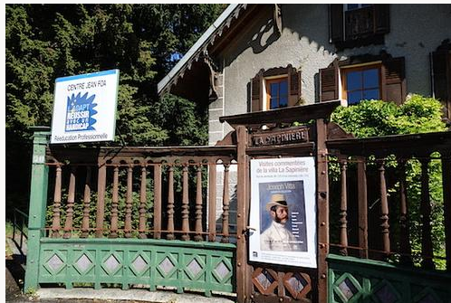
Fig. 26, La Sapinière: Gate house. [larger image]
