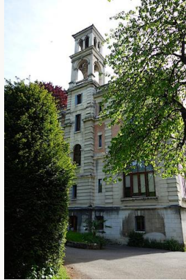
Fig. 27, La Sapinière: Jean-Camille Formigé, Rear façade. [larger image]
