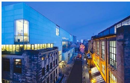
Fig. 13, Steven Holl, Reid Building and the Mack before the fire.
