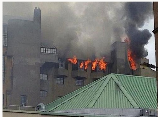
Fig. 9, Flames coming out of the Hen Run on the south façade. [view image & full caption]
