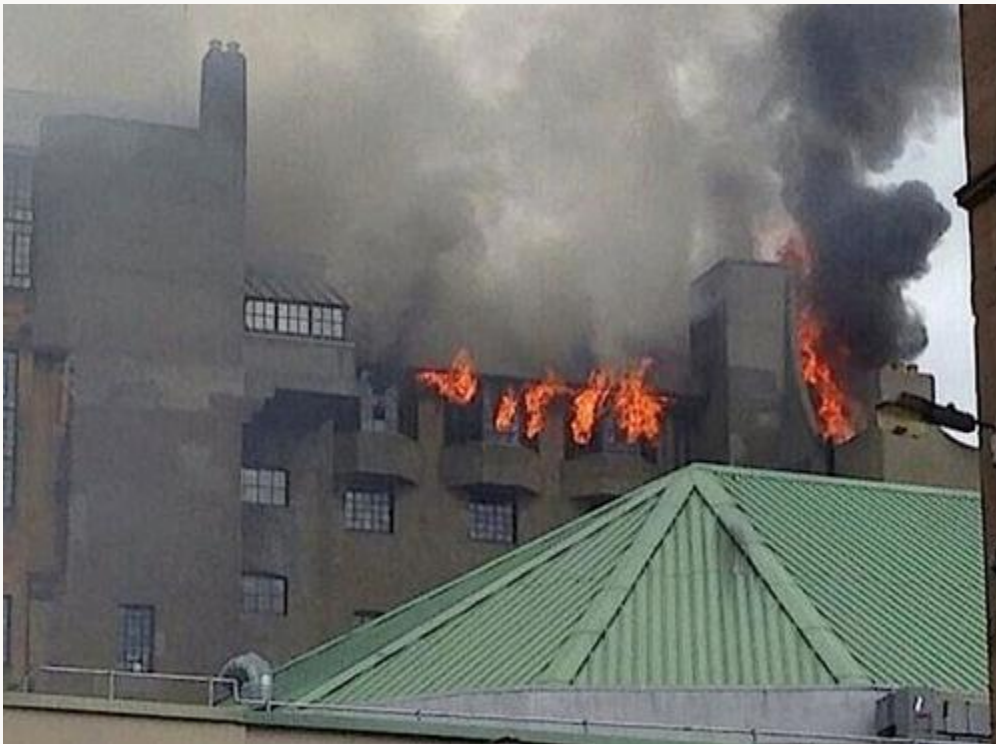
Fig. 9, Flames coming out of the Hen Run on the south façade. Public Domain. [return to text]
