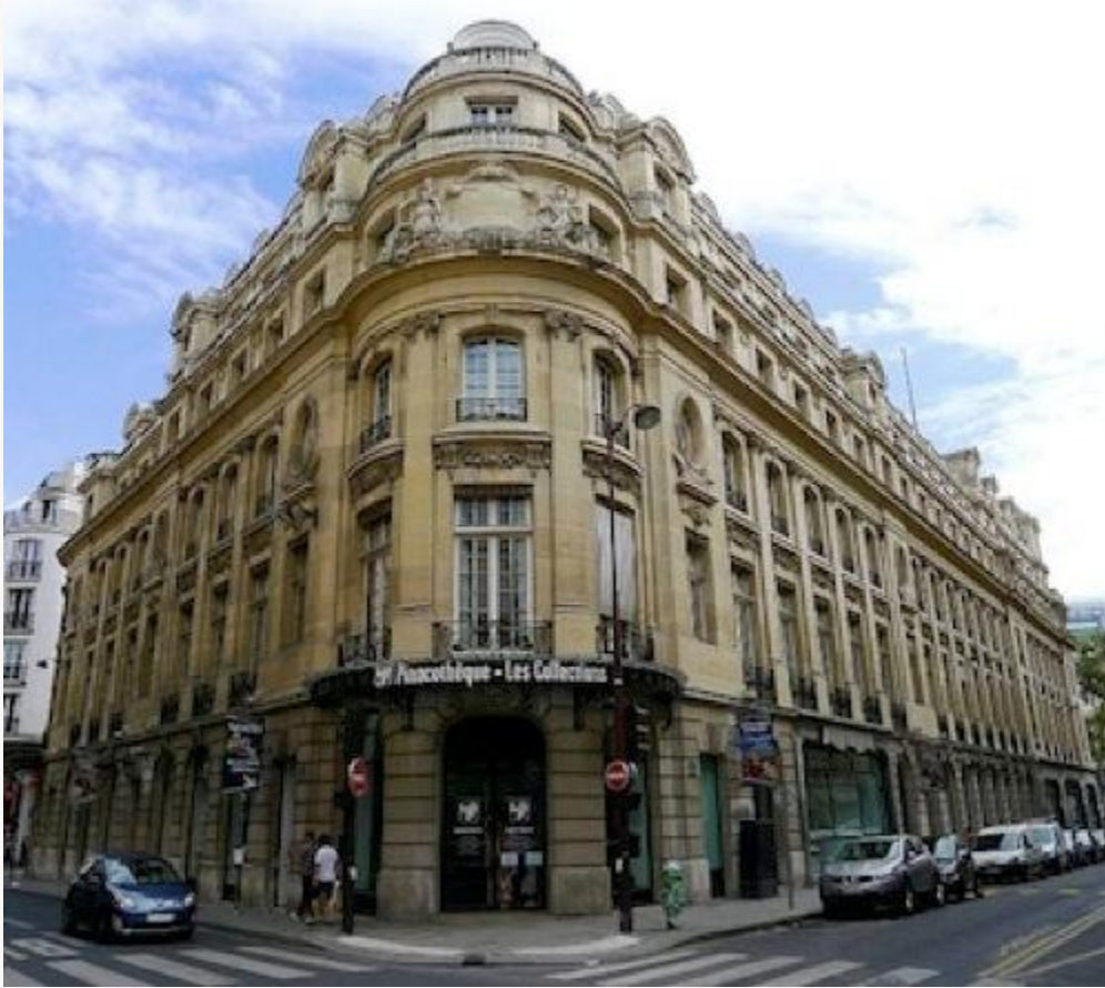
Fig. 1, View of exterior of Pinacothèque de Paris. [return to text]
