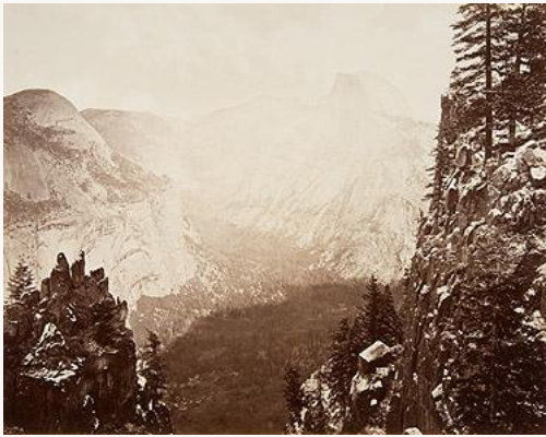
Fig. 5, Eadweard Muybridge, The Domes, Valley of the Yosemite, from Glacier Rock, California , 1872.
