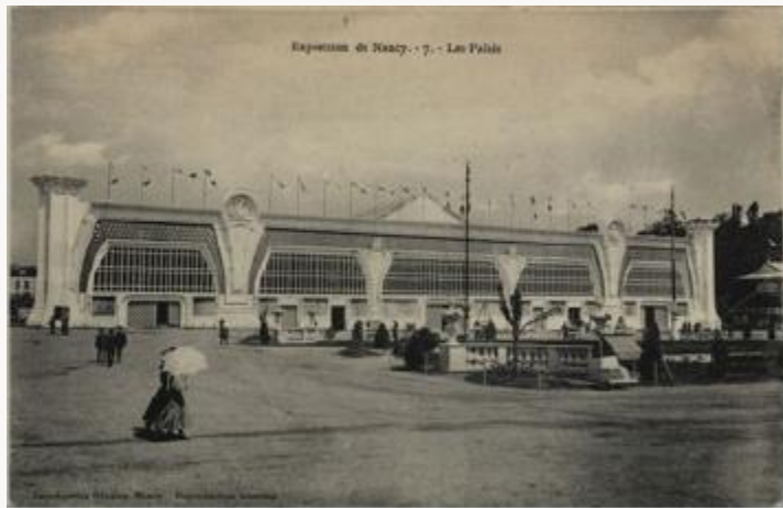
Fig. 20, Louis Lanternier and Eugène Vallin, Pavilion of Mines and Metallurgy, Exposition Internationale de l'Est de la France, Nancy, 1909. Postcard, collection of the author. [return to text]
