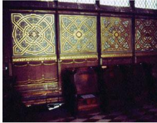
Fig. 24, Detail of painting below window in the north transept, Chapel, St. Michael's Abbey, Farnborough
