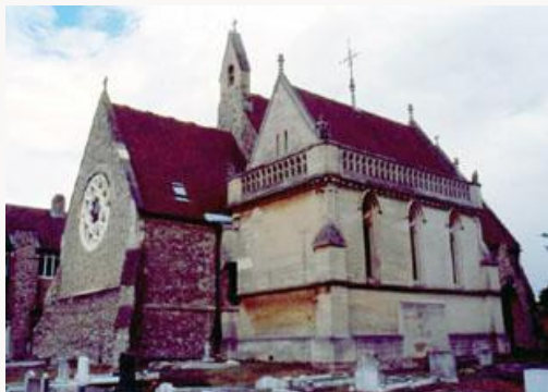
Fig. 2, Addition to St. Mary's Church, Chislehurst
