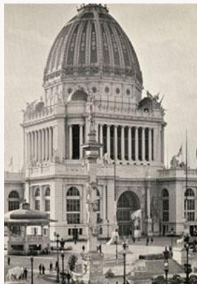
Fig. 3, The Administration Building, from the South East , 1893. Photograph by William Henry Jackson, reproduced in Jackson 1894 [larger image]
