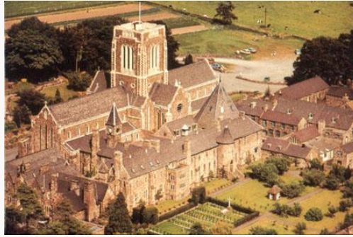
Fig. 8, The south front of Mount Saint Bernard Abbey, ca. 1990. Pugin completed the western portion of the church (left of the tower) and the cloister area attached to it. Between 1934 and 1939 architect Albert Herbert of Leicester added the transepts, tower, and eastern nave. Pugin's son, Edward Welby Pugin, completed the octagonal chapter house south of the tower transept in 1860. (Courtesy of the monks of Mount Saint Bernard Abbey) [larger image]
