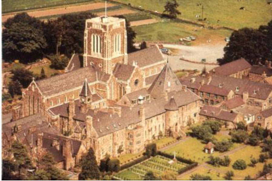
Fig. 8, The south front of Mount Saint Bernard Abbey, ca. 1990. Pugin completed the western portion of the church (left of the tower) and the cloister area attached to it. Between 1934 and 1939 architect Albert Herbert of Leicester added the transepts, tower, and eastern nave. Pugin's son, Edward Welby Pugin, completed the octagonal chapter house south of the tower transept in 1860. (Courtesy of the monks of Mount Saint Bernard Abbey) [return to text]
